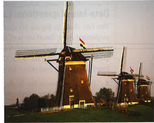
▲ Figure 9 During the industrial revolution renewable sources of power including wind were replaced with power generated by burning fossil fuels
